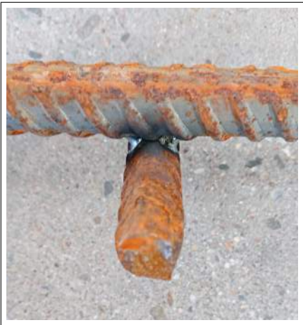
(d) Picture showing welded connection between rebars.
