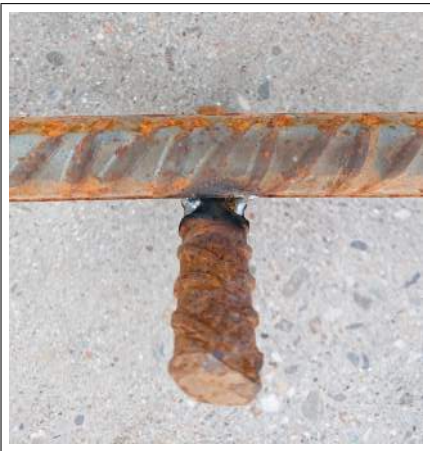
(c) Picture showing welded connection between rebars.
