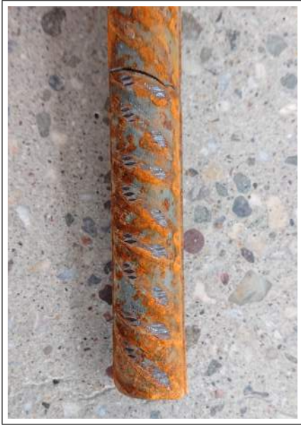
(a) Crack at gripping area. Machine jaw marking just over ribbing area.
